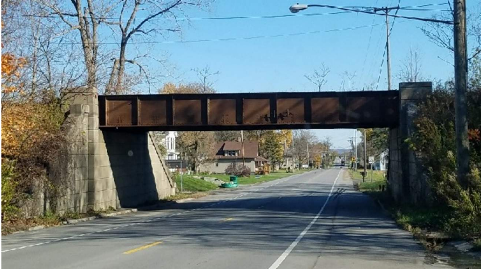
Photo 8 – Existing Erie Lackawanna Railroad Bridge looking east
